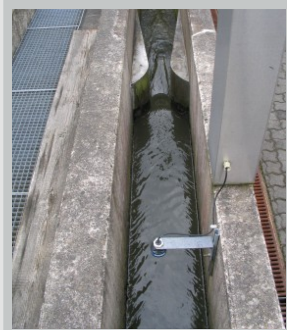
Venturi flume measurement in discharge
