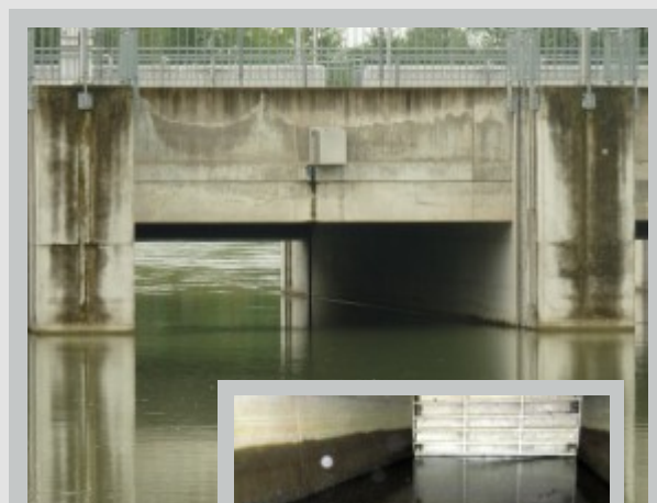
Polder gate and installed sensors
