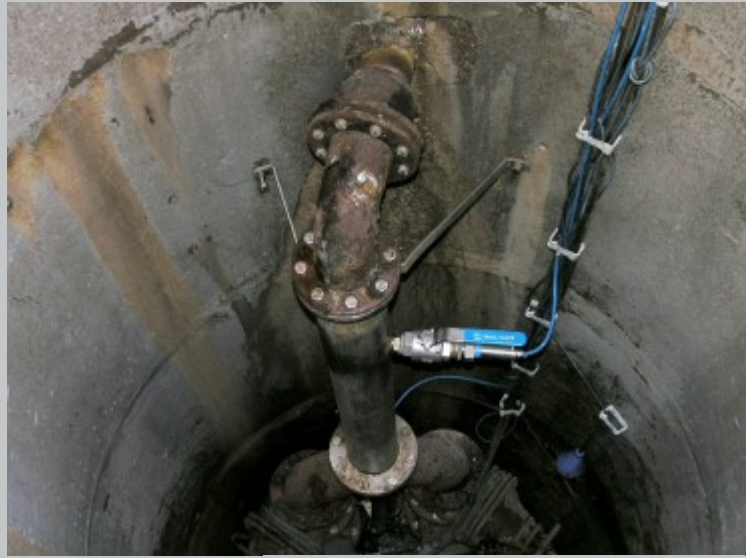
Pump shaft with built-in measurement system
