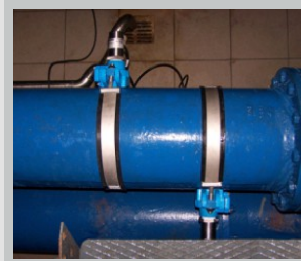
Filling and drain pipe with installed sensors
