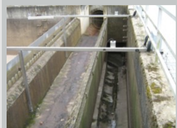
Overflow sill as trough in basin
