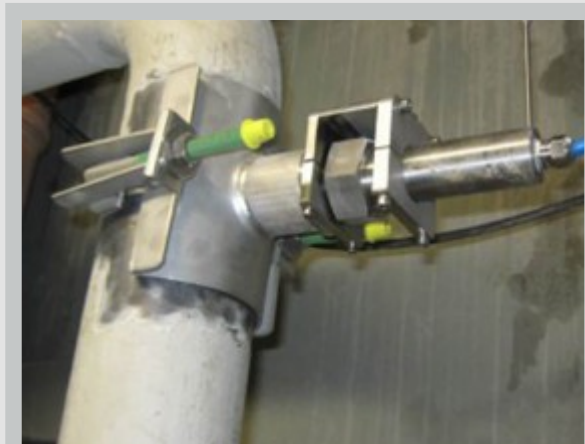
Installed sensor with tapping saddle
