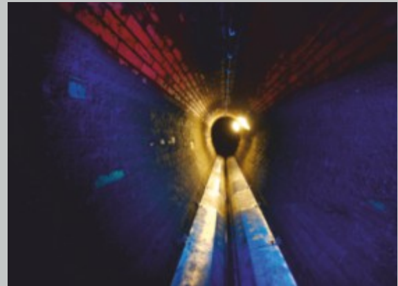
Wastewater heat exchanger (Photo: ECO.S)
