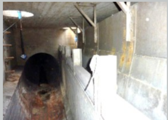
Stormwater overflow sill
