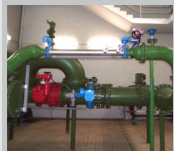
Nighttime supply measurement point in bypass pipeline
