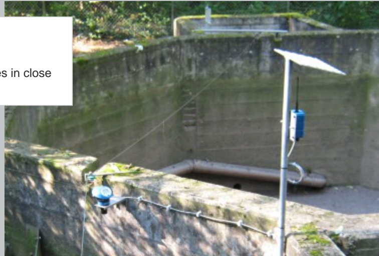
Tank with installed level sensor and data logger
