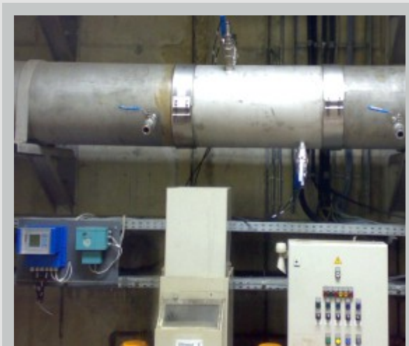
Sensors installed in pipe line
