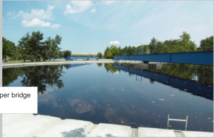
Secondary clarifier with scraper bridge
