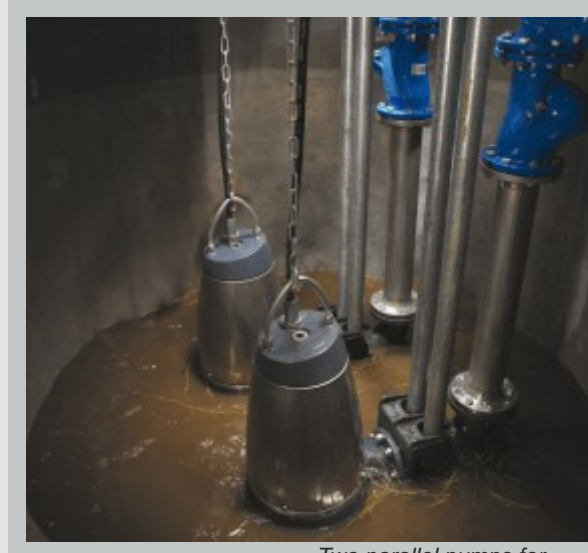
Two parallel pumps for pressure boost
