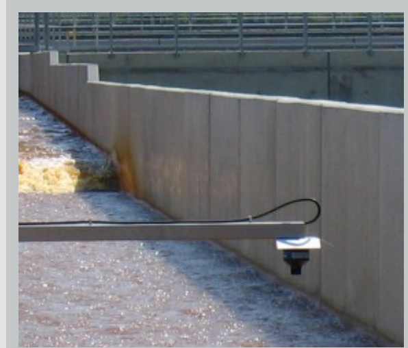
Measurement point with level sensor
