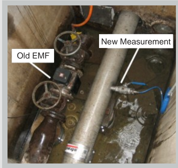
Top view on measurement place
