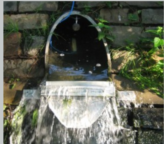
Discharge pipe with impoundage shield
