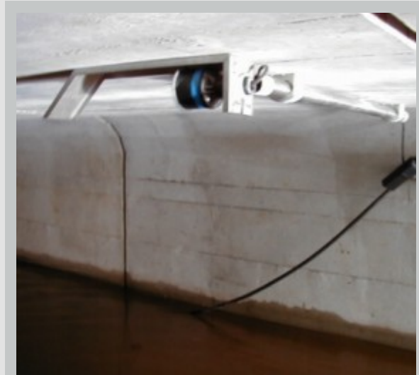
Ultrasonic level measurement with tilted mirror
