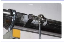
Pipe clamp for explosion-hazard areas attached to a stainless steel pipe (StSt)
