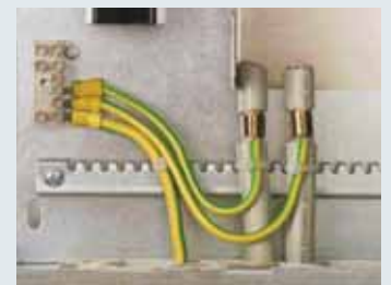
Shield connection with SA KRF
